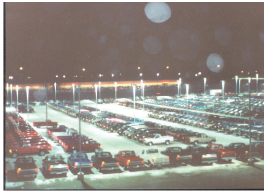
A lighter, brighter concrete parking area provides an inviting entranceway to you business.
