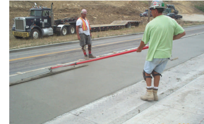
Concrete was given a coarse broom texture finish.
