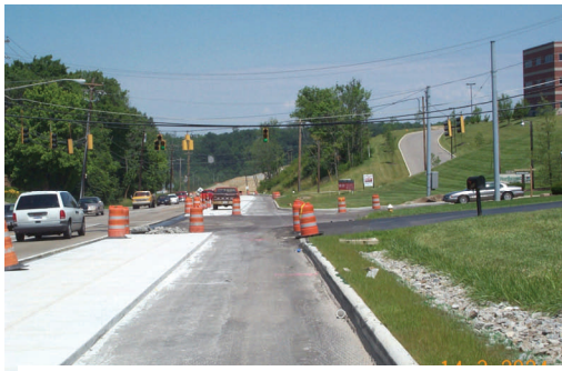
The speed lane was placed first with the curb lane to follow.
