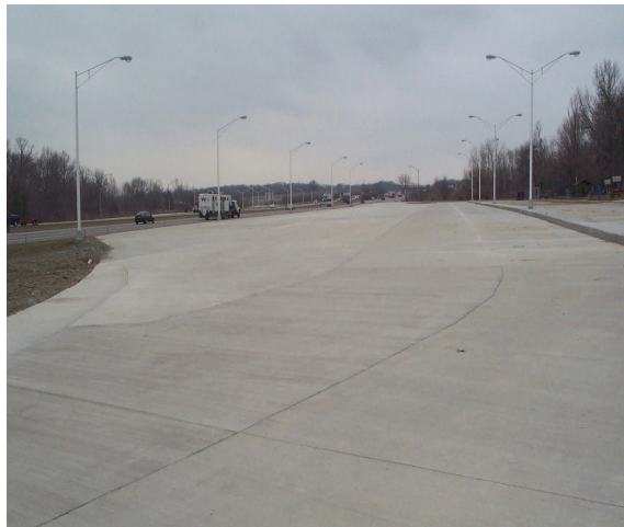
Concrete provides a lighter, brighter, safer rest area for ODOT and Butler County.
