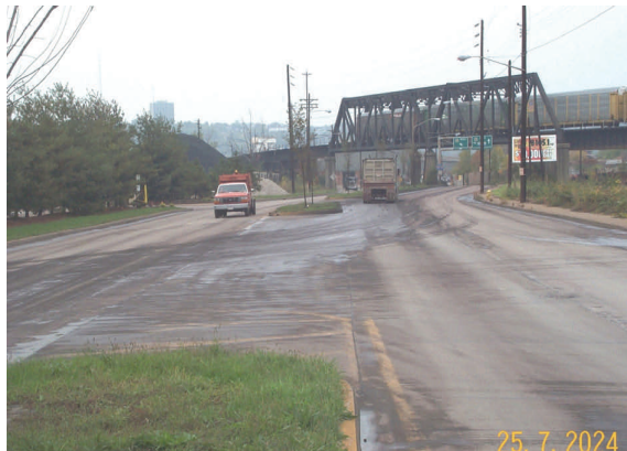
View westbound on Mehring Way toward the C&O Railroad bridge.
