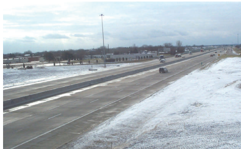
Southbound view from the SR 41 overpass.
