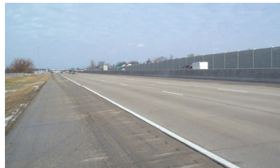
12-foot travel lanes with a 16-foot
