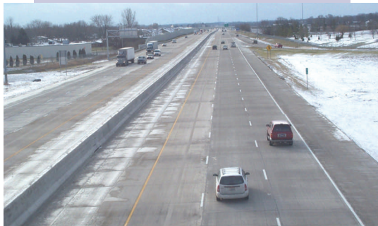
Durable, long-lasting concrete carries the loads today and tomorrow
