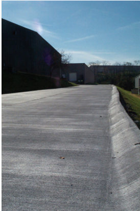
Entrance to the receiving area of N. Kentucky industrial complex
