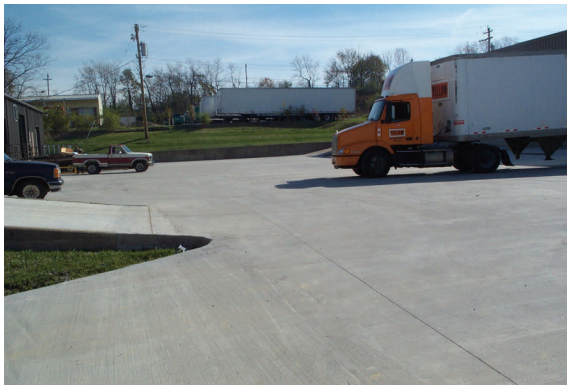
Just days after completion, this lot is handling traffic.
