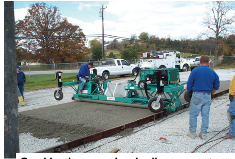
Combination screed and roller compactor
