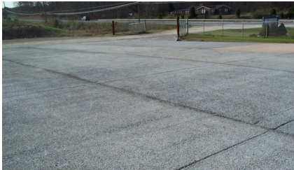
Pervious concrete parking lot will handle water runoff.
